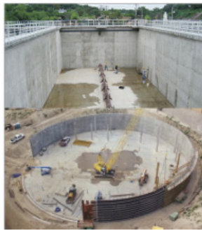
Concrete tank in water treatment plant / Water storage concrete tank.
