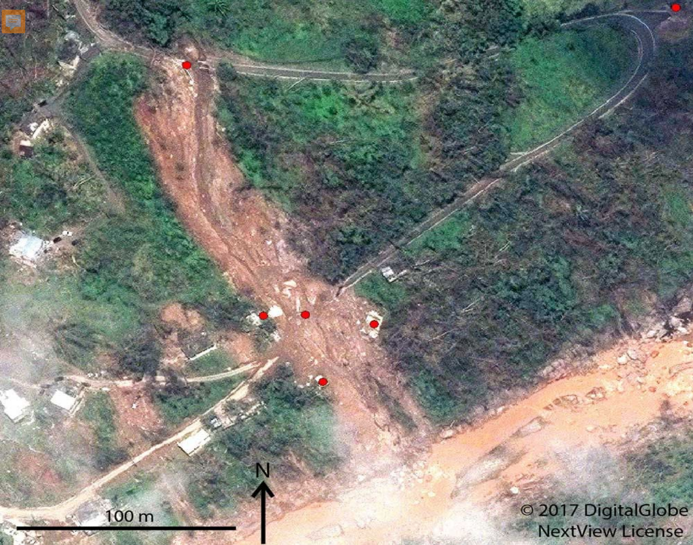
Road damaged by Mudslides
