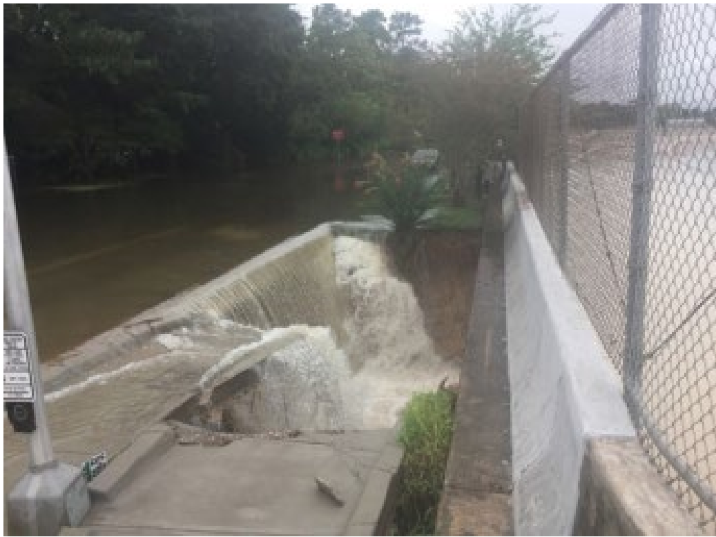
Damage of the walkway slab on Beltway 8 (left photo courtesy a resident in the area, August 27, 2017, and right photo courtesy of a construction worker on site
