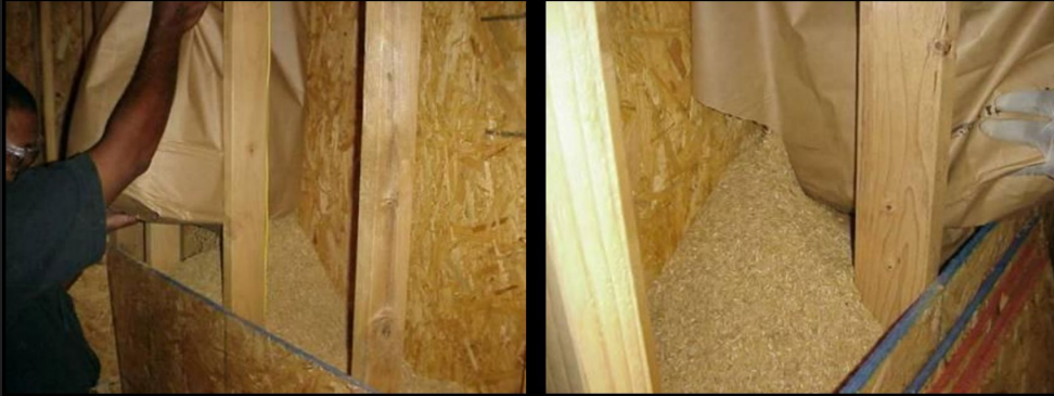
Figure 2: Rice Hull insulation construction
